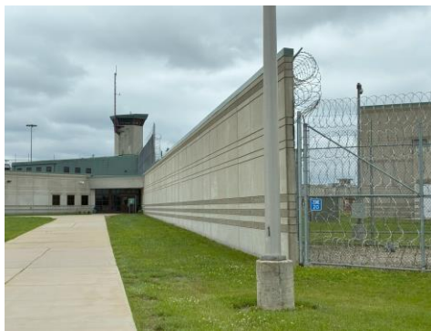
Photograph of building behind barbed wire within Miami Correctional Facility, taken on June 22, 2026
