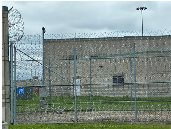
Photograph of building behind barbed wire within Miami Correctional facility, taken on June 22, 2026
